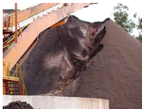
Figure 1. Failure of a pellet feed stockpile at the port of Vitoria.
